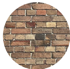
XBR1 - Existing brickwork, type 1
