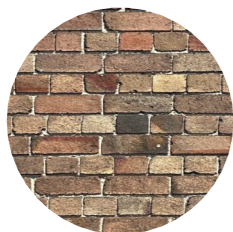
XBR1 - Existing brickwork, type 1
