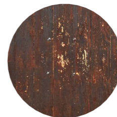
XTPD - Existing Timber Panelled Door
