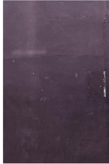
XBRRP - Existing brickwork, render paint finished
