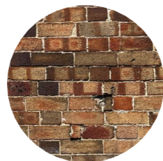
XBR2 - Existing brickwork, type 2
