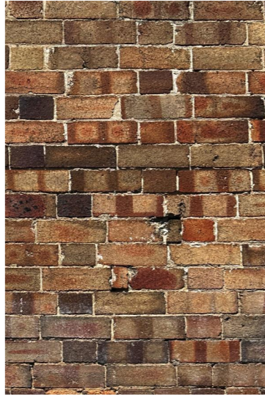
XBR2 - Existing brickwork, type 2
