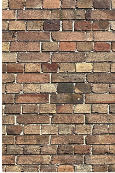
XBR1 - Existing brickwork, type 1
