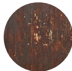
XTPD - Existing Timber Panelled Door
