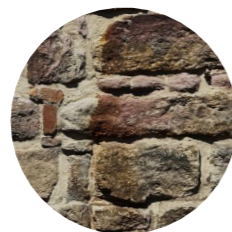
XSTW - Existing sandstone wall
