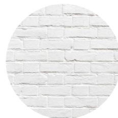
XBRRP - Existing brickwork, render paint finished
