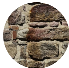
XSTW - Existing sandstone wall
